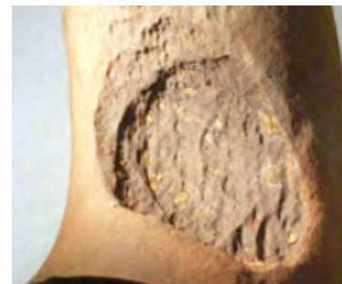
Figure 4: Field recovered chain links (76mm diam.) after surface cleaning showing highly varied local corrosion.
