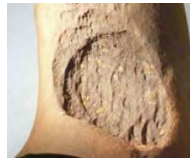
Figure 4: Field recovered chain links (76mm diam.) after surface cleaning showing highly varied local corrosion.
